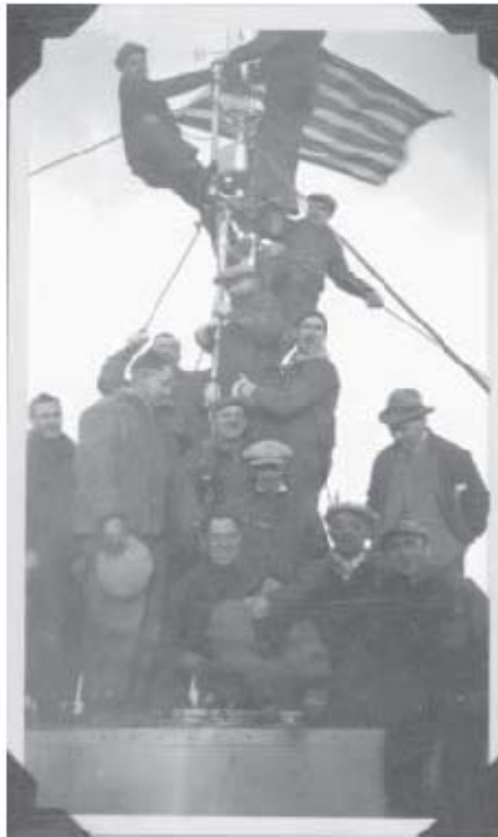
Workers raise the topping out flag on the completed mooring mast of the Empire State Building (March 18, 1931).
